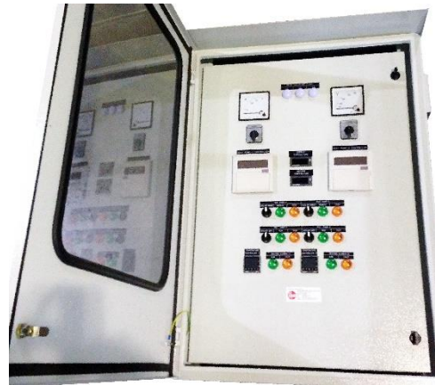
Outdoor Enclosure Panel (Double Door, IP54)
