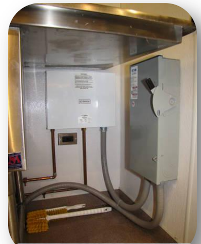
Eemax Electric Tankless Water Heaters take up very little space and can be mounted right at the point of use.
