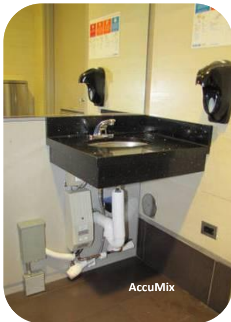
ProAdvantage Units Eemax ProAdvantage and AccuMix units are ideal for placement under hand washing sinks.
