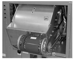
provide quiet and efficient airflow. The blower sheave is secured by an "H" bushing which firmly secures the pulley to the blower shaft for years of trouble-free operation. The "H" bushing allows for easy removal of the blower pulley from the shaft, as opposed to the use of a set screw, which can score the shaft, creating burrs that make blower-pulley removal difficult.
