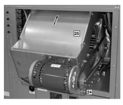
provide quiet and efficient airflow. The blower sheave is secured by an "H" bushing which firmly secures the pulley to the blower shaft for years of trouble-free operation. The "H" bushing allows for easy removal of the blower pulley from the shaft, as opposed to the use of a set screw, which can score the shaft, creating burrs that make blower-pulley removal difficult.
